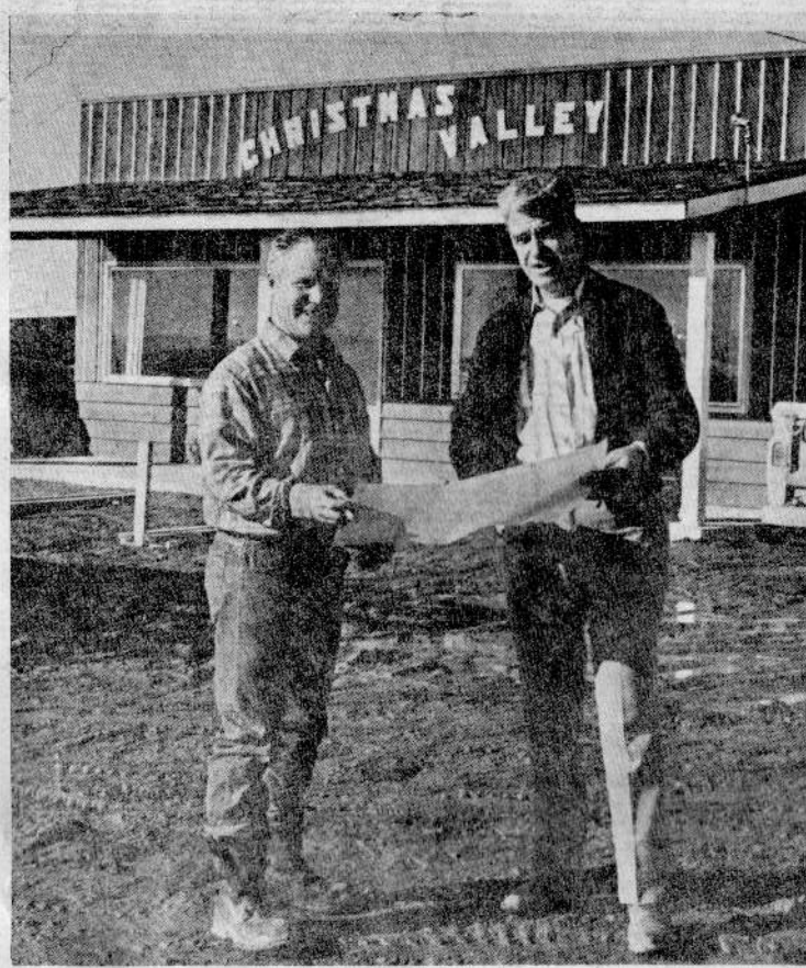
Responsibility for the development and building program in Christmas Valley rests with Warren W. Morton, left, Project Manager, and Harold Boyer, Construction Superintendent. And what they've done in just a few short months has been nothing short of sensational! But they claim they haven't really gotten started yet, just wait until they get into high gear. It promises well for the future of the Valley.
